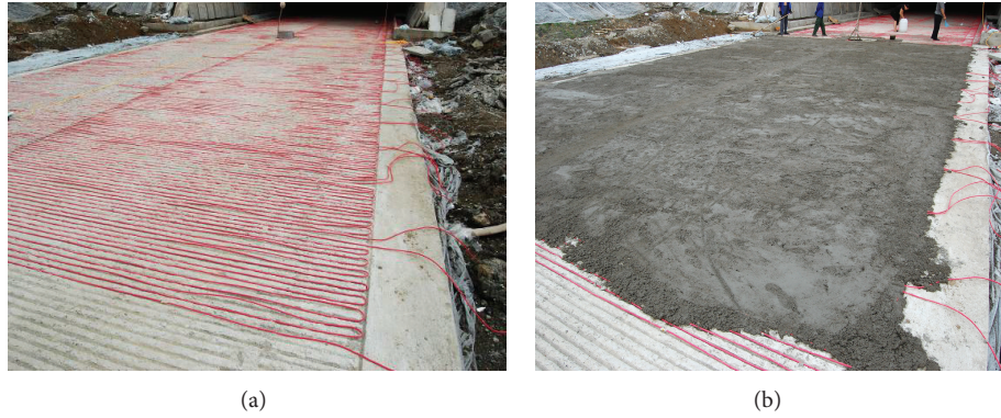
FIGURE 8: On-site construction of electric heat tracing system.
